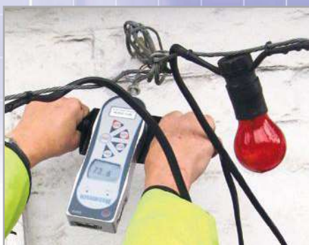
Pull test on anchorage points
